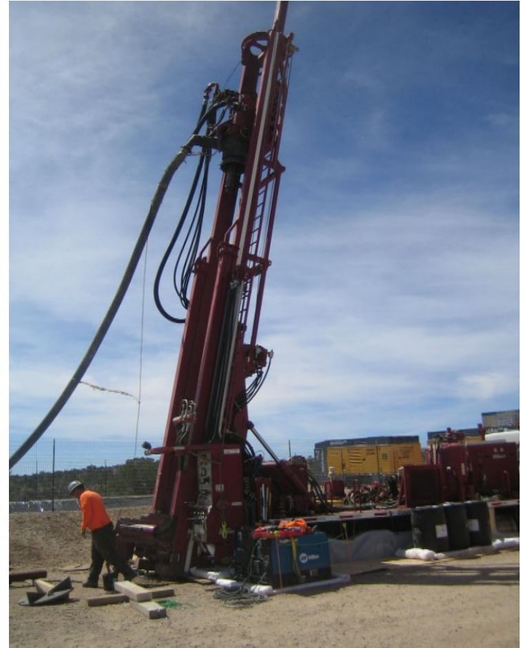
Angled Drilling at Chromium Project
